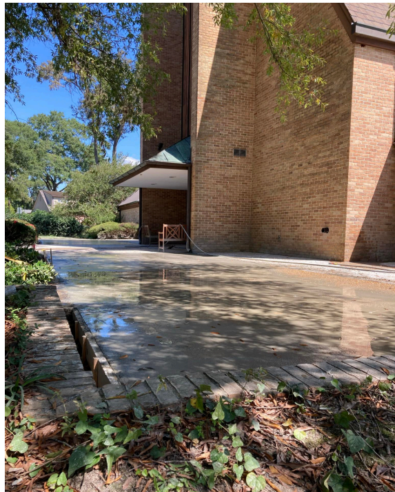
A NEW PATIO WAS POURED IN SEPTEMBER
