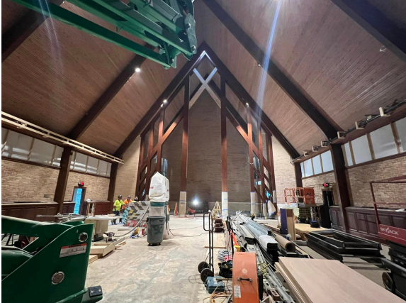
BRICK WORK IS COMPLETE
